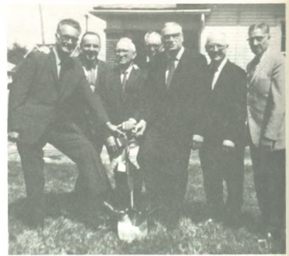
ACTUAL construction is now under way for New Castle (Ind.) First Church. Contractors estimate it will be completed before the end of the year. The building, which is estimated to be a $200,000 structure, will be contemporary in style. The new sanctuary will have a normal seating capacity of 350 with overflow facilities to accommodate another 250 persons. Included in the new plan are administrative offices, additional educational facilities, and remodeling of the present two-story Sunday school annex. Long-range plans include construction of a fellowship hall and all-purpose building. Morris Chalfant is pastor. Pictured left to right, Mayor Paul Osborne, Morris Chalfant, Building Chairman Philip Greer, E. B. Caldwell, District Superintendent Rev. Ross Lee, Dan Torgrinsson, and Roger Garner.
