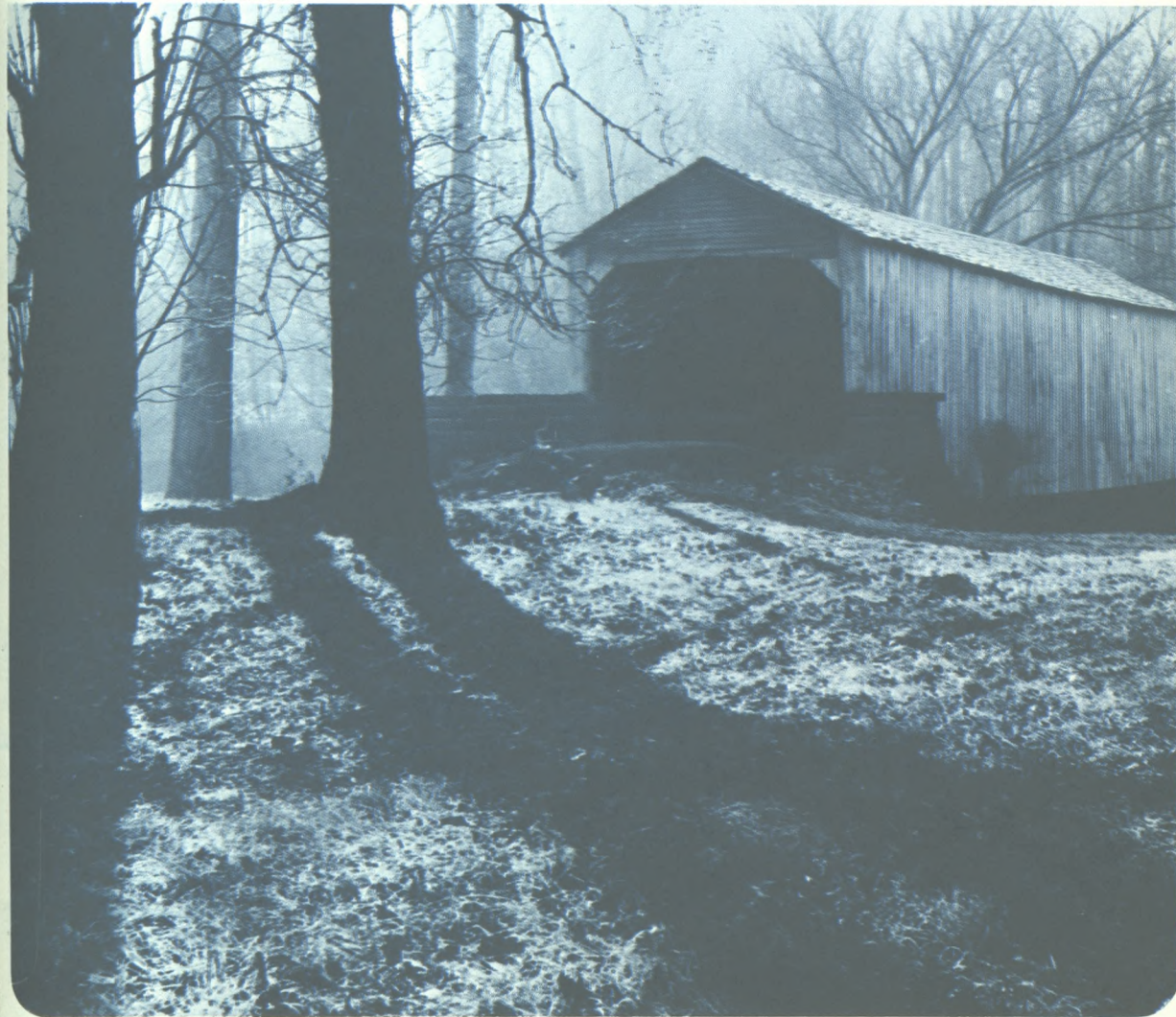
Covered bridge near Chester, Illinois
