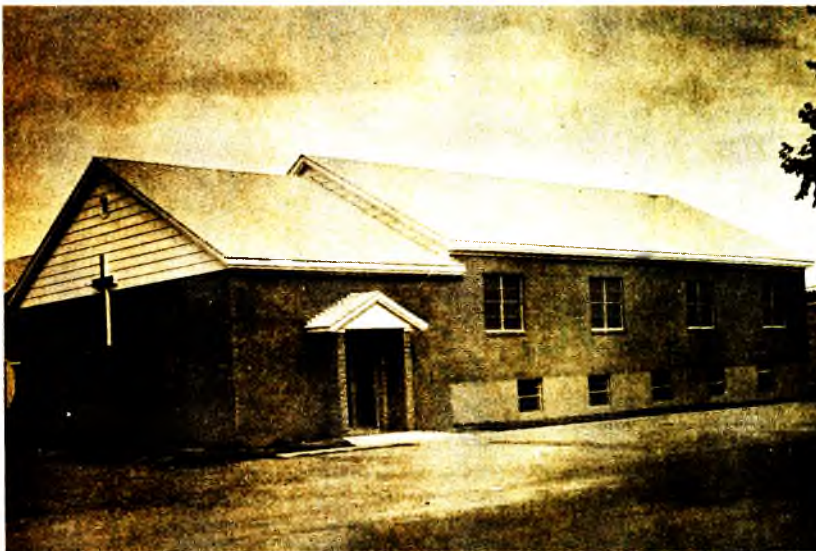
OKLAHOMA CHURCH REMODELED —Rev. Jerald Locke, Northwest Oklahoma District superintendent, spoke at the recent dedication services of the Watonga, Oklahoma, church. A total of $23,000 was spent on enlarging and remodelling the church, according to Pastor Roy L. Bickford.
