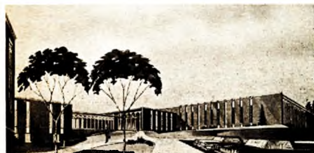
NEW LIBRARY BUILDING
