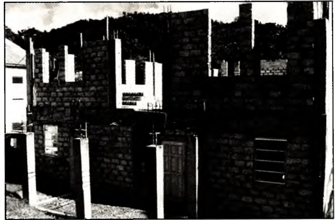
Construction of the new Castries Church of the Nazarene
