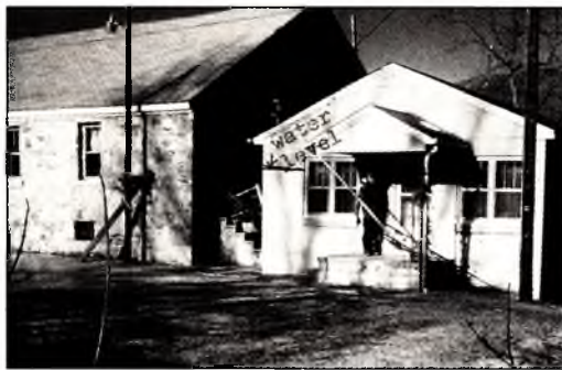
The line on this photograph shows the waterline at the annex of the Marlinton, W.Va., Church of the Nazarene caused by flooding in January.
