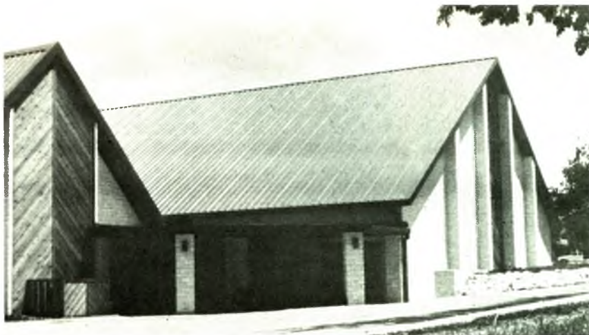
The South Austin, Tex., church dedicated its new sanctuary May 13. This addition will seat 400 with an overflow area in the balcony. Cliff Hoerling, a layman from the church, volunteered his services as general contractor. Since its relocation 13 years ago, the South Austin church has grown from a congregation of 60 to 250 and has a Christian school for K—9th grade and a day care with 300 students enrolled. The 5,200 sq. ft. structure was built at a cost of $310,000, with an indebtedness of $192,000. General Superintendent Orville W. Jenkins gave the dedicatory message, with Dr. James Blankenship, superintendent of the San Antonio District, assisting. Rev. Randall Wyles has pastored the church since 1972.
