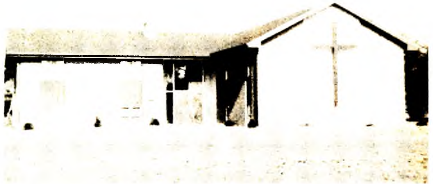
The Bristol, Ind., church dedicated their new combination church and parsonage on Sunday, June 10. Dr. Bruce T. Taylor, district superintendent, was in charge of the dedication service. Rev. Joseph F. Chapman is pastor. The structure was built at a cost of $120,000, with much donated labor from the Men in Mission group from North-eastern Indiana District. The building is located on five acres of land and the value of the property exceeds $200,000.
