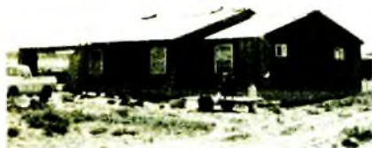
The parsonage nearing completion
